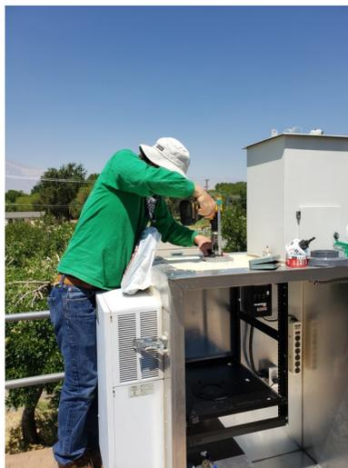
Right: The outdoor enclosure after the first stage of modification was completed, ready for weather sealing, and then the replacement monitor, on the monitoring platform, next to the PM<sub>10</sub> monitor.
